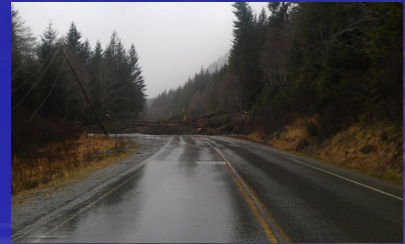
Landslide on the Klawock-Hollis Highway, courtesy of state troopers.
