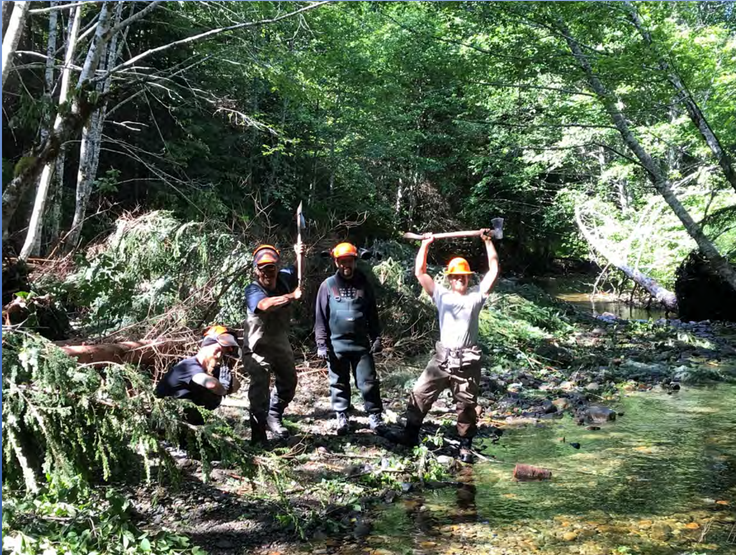
Upstream HNFP crew – 2 hand tool sites installed. 7 equipment sites installed downstream.
