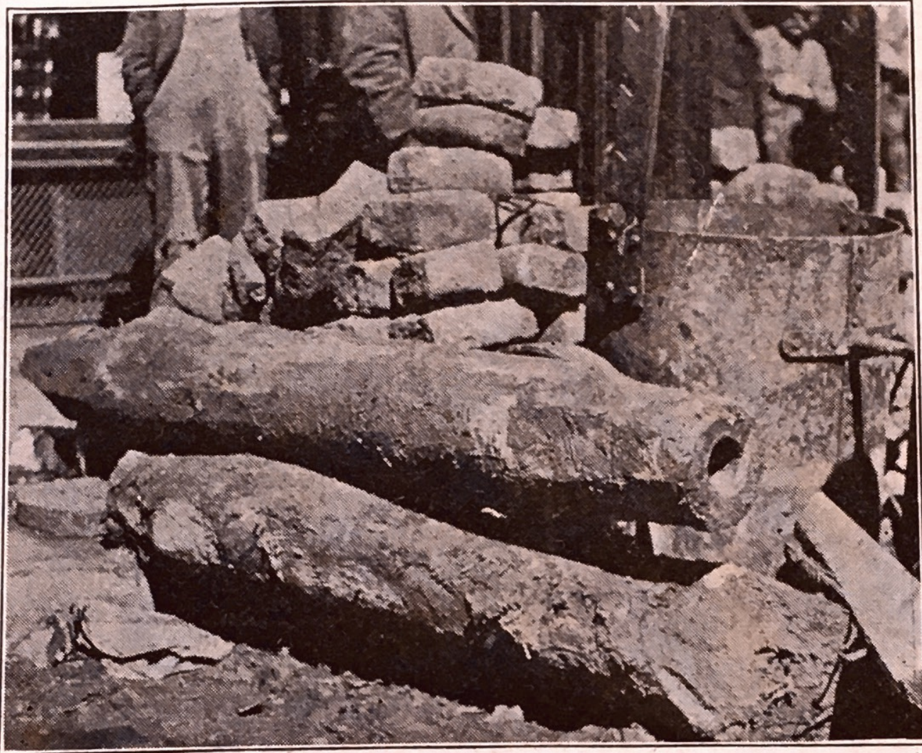
CHESTNUT WATER PIPES LAID IN BOSTON 125 YEARS AGO AND STILL IN SOUND CONDITION.
