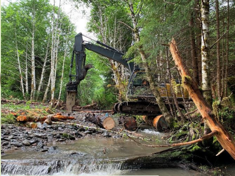
Protecting banks during access with logs
