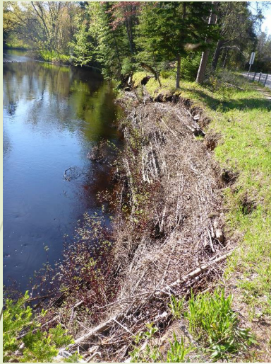
Sturgeon River, Michigan 1 year after construction
