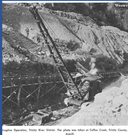
Dragline Operation, Trinity River District. The photo was taken at Coffee Creek, Trinity County, in 1940. Photo courtesy of Western Consolidated Industries.
